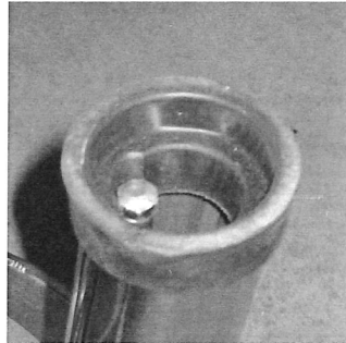
Figure 6: Tightening leg bolts and fitting plastic foot.
